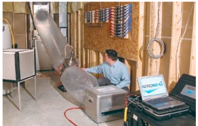
AeroSeal – duct sealing from the inside.
